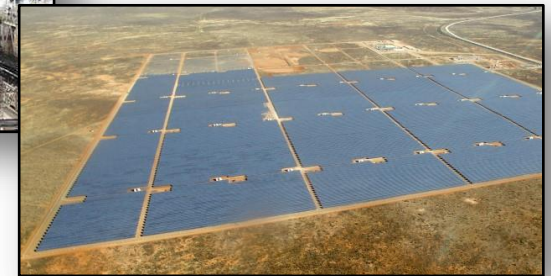
2013: Scatec Solar finishes South African 75 MW project
