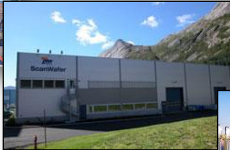
1994: Scanwafer established in Glomfjord Production capacity ~75 MW
